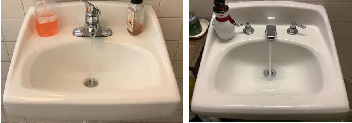
Typical Restroom Sinks
