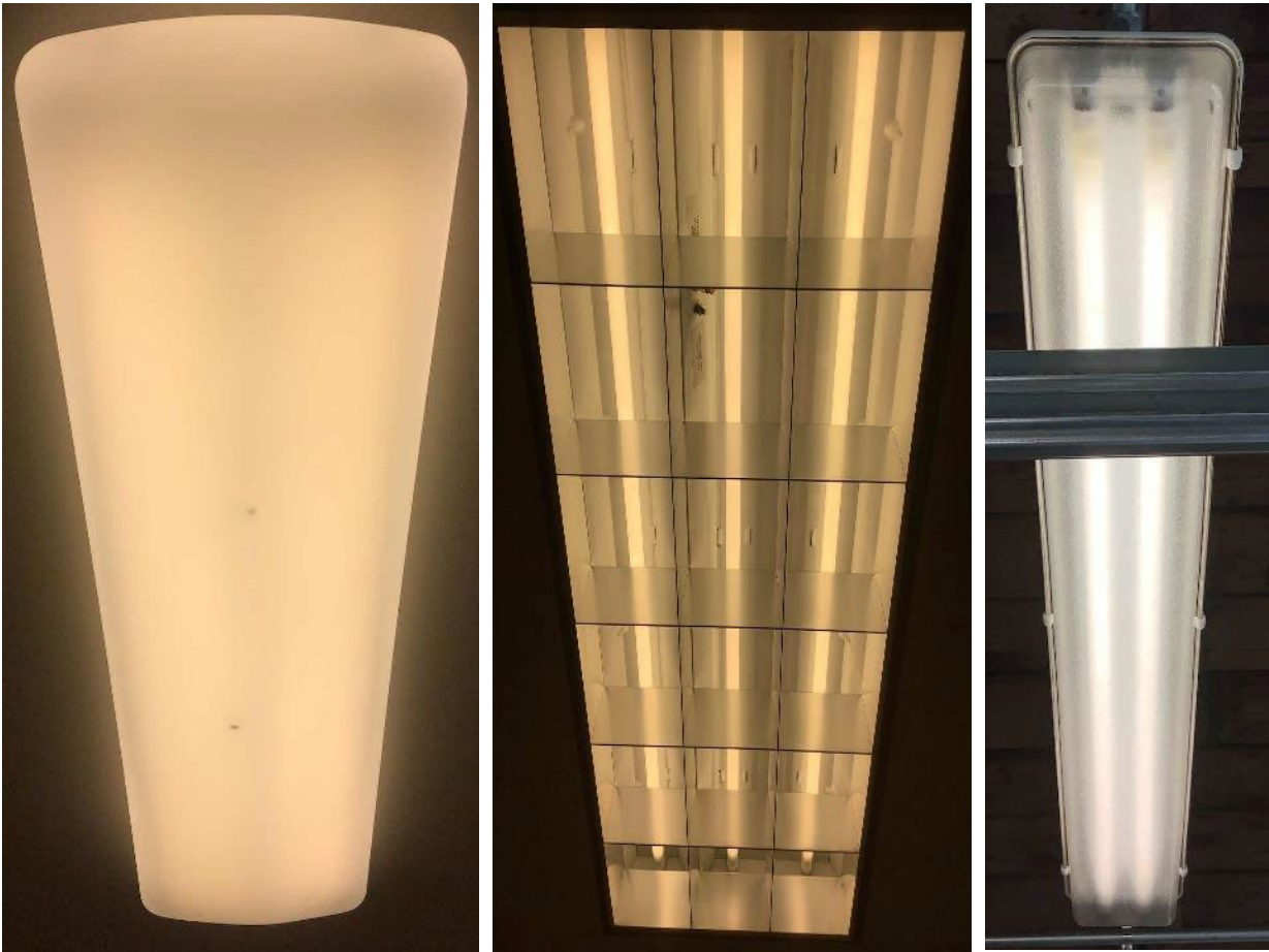
Fluorescent T8 Fixtures
