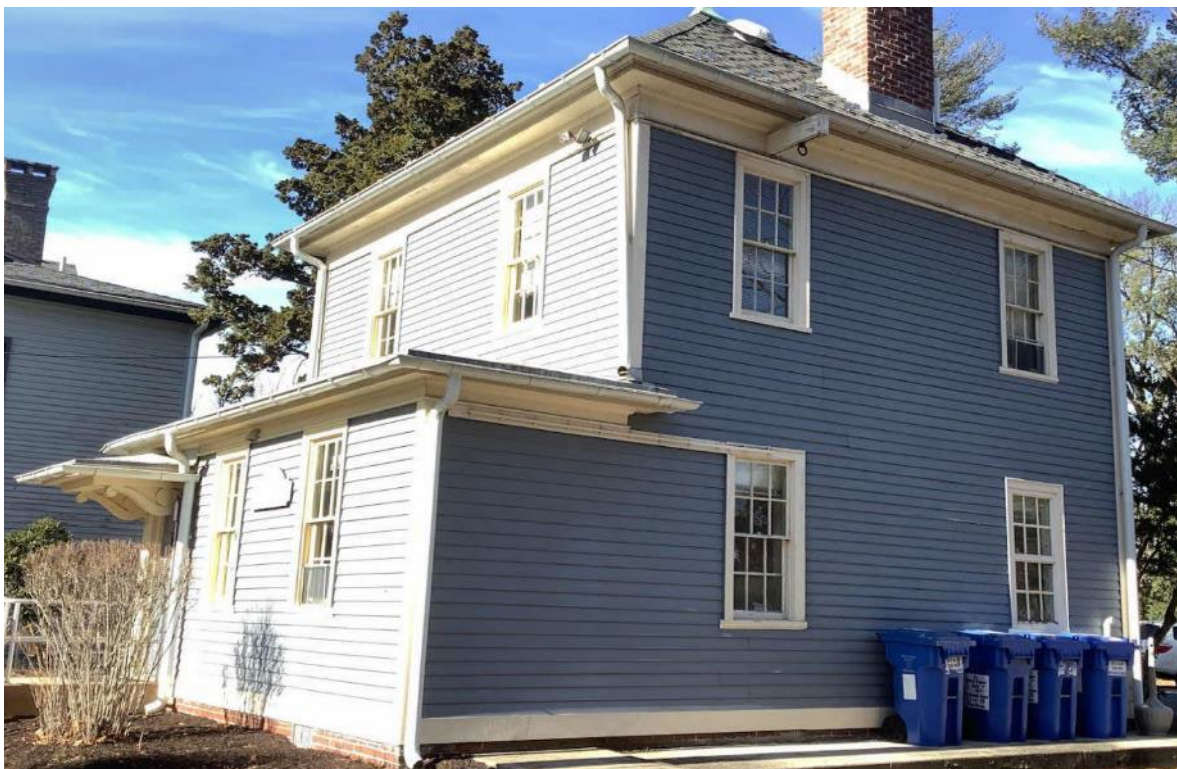
Building Walls – Carriage House
