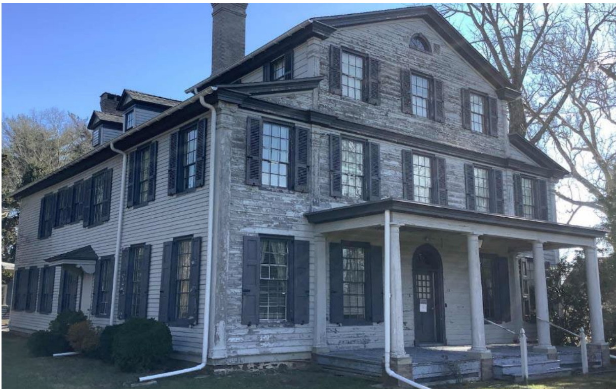
Building Walls – Fenwick Manor
